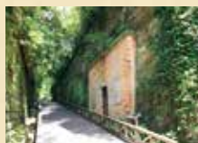
Cut Passage (Fortress site) The treasured brickwork of old fortress facility with the barracks, ammunition depot, and more.
